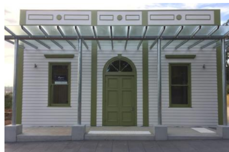
The recently restored Glenlyon Hall.
