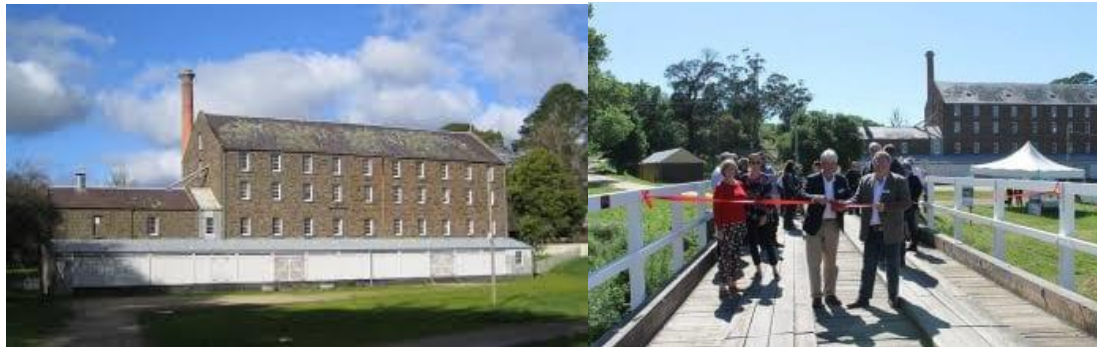
Andersons' Mill, Smeaton and opening of the restored bridge (Source: Hepburn Shire Council)
