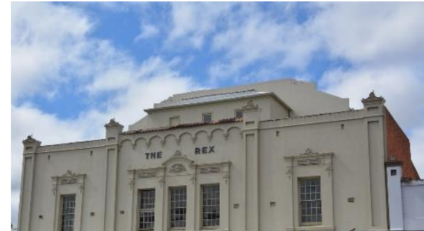
Council recently purchased the locally significant (former) Rex theatre to be converted to the shire's new administration centre. (Source: Hepburn Shire Council)
