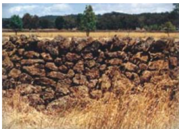
Dry stone wall, Hepburn Shire Photo: Raelene Marshall
