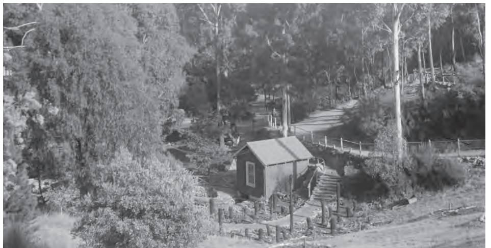
Photograph 13: The pump shed from the Lake Daylesford dam wall embankment
