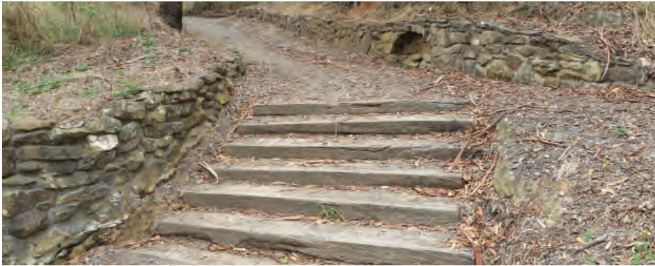
Photograph 3: Existing non-DDA compliant stairs to the east of the Central Springs
