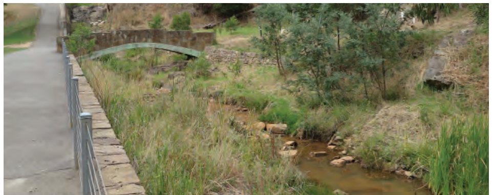
Photograph 4: Looking upstream along the Creek from the stand of deciduous trees
