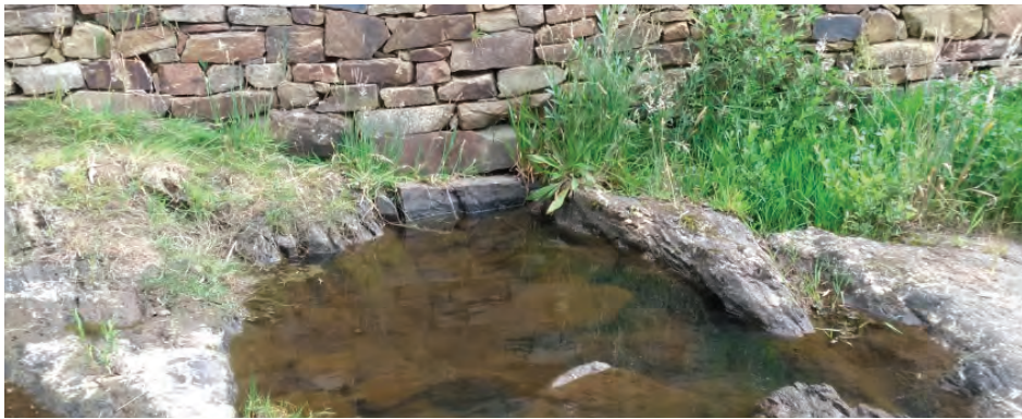
Photograph 5: The Cascades feature with built stone retaining wall behind.
