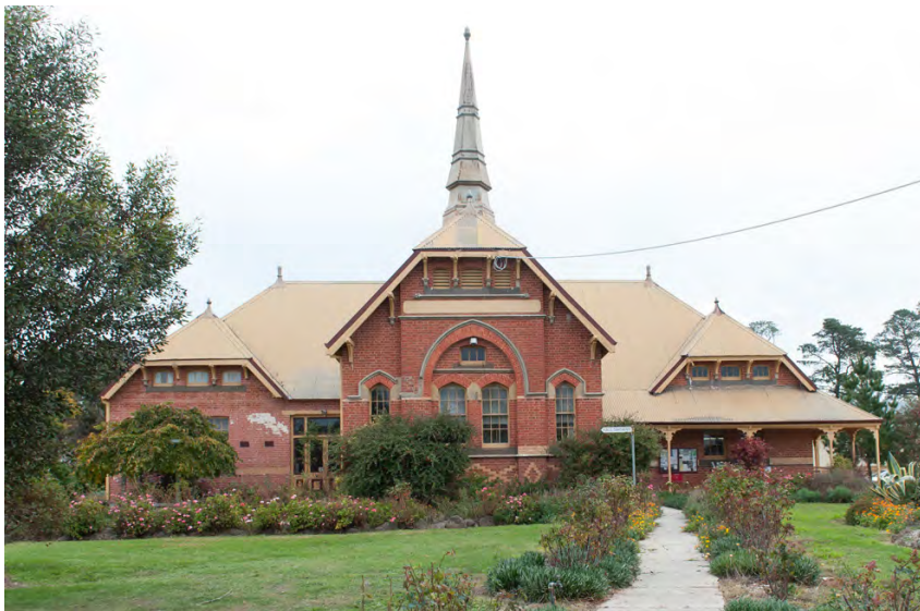
Front entrance facing Bailey Street, Clunes.
