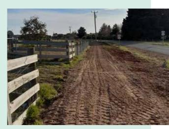
▲ Works started on the second and final stage of the Daylesford-Coomoora walking trail. The 1.5m wide path was constructed from recycled crushed concrete.
