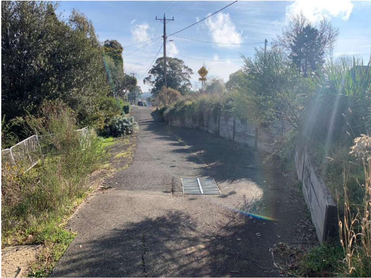
Figure 10 Looking north from Goldfields Track onto Main Road and existing widening to Goldfields Track (RHS)
