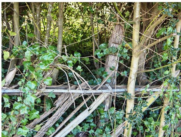
Remnant fencing showing timber pickets, timber posts and metal strip (possibly similar to 'iron hooping' referred to in History 1906
