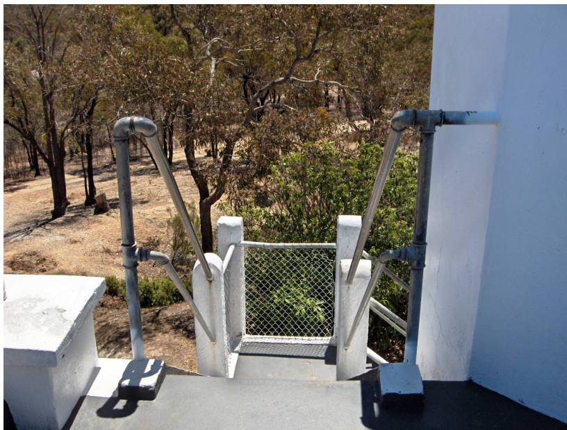
Figure 63: Detail of retaining fence at top and on landing of Pioneers' Memorial Tower, Maryborough [Lee Andrews, 2006]
