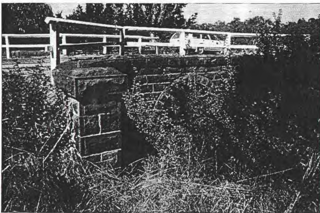
Basalt culverts, constructed at Amherst in the late 1850s, are now some of the earliest public works surviving in the Shire.
