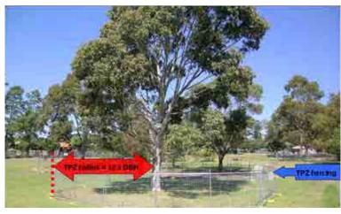
Figure 3: TPZ fencing is erected around retained trees prior to site works
