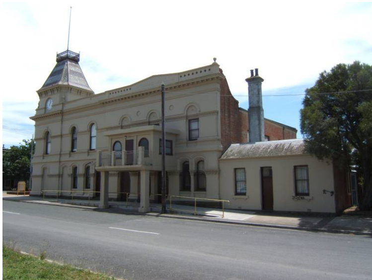
2 Water St – Attached cottage at rear of Creswick Town Hall
