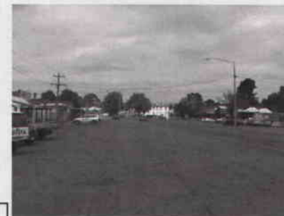
Wide Street crossing at northern aspect of Albert Street, Creswick.
