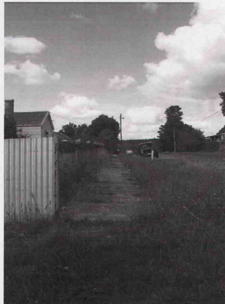
Hall Street Footpath, Creswick. Maintenance required.
