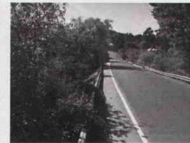
Bleakley Street-current access for pedestrians over bridge at Lake Daylesford.
