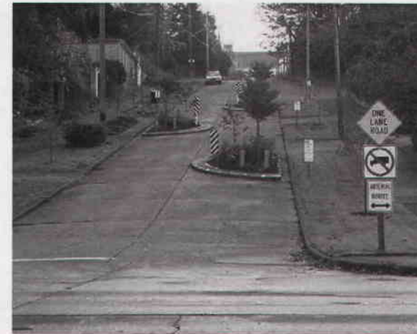
Chicane provides traffic calming in a one way street
