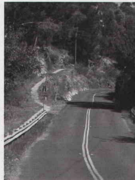
Pathway to Hepburn Primary School is steep and requires some railing to protect from the edge of the incline.
