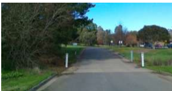
Existing Culvert on Moore St
