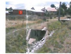
m- view of drain at the front of the subject site
