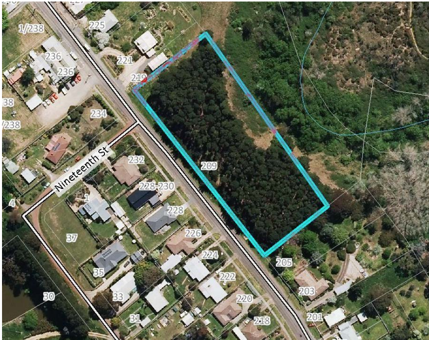
Aerial Photo (Prior to Pine Tree removal)
