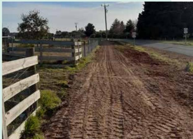
▲ Works started on the second and final stage of the Daylesford-Coomoora walking trail. The 1.5m wide path was constructed from recycled crushed concrete.
