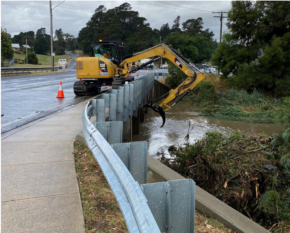
Image: Clearing debris out of Creswick Creek following the storm event
