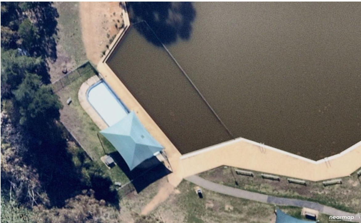
Figure 16: Aerial view of Calembreen Park Toddler Pool
