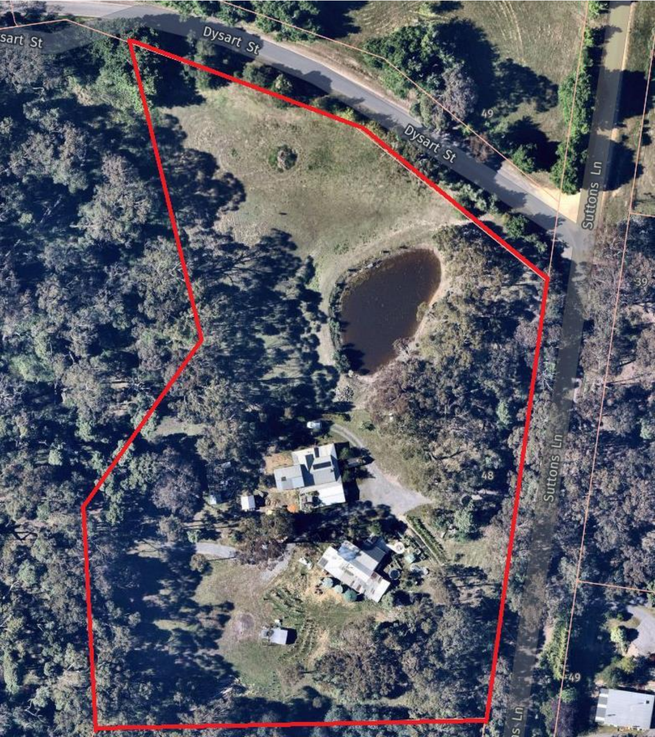
FIGURE 3 EXISTING CONDITIONS AIR PHOTO
