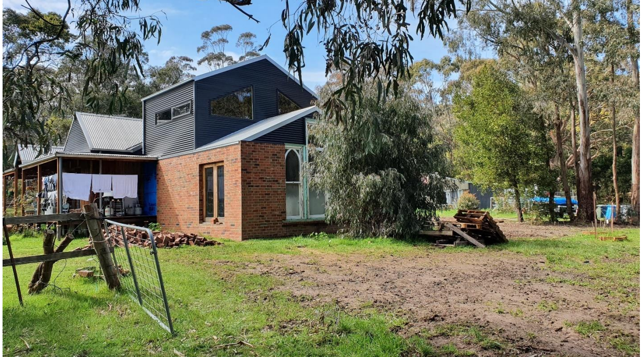
Photo 2 Looking south east to the existing dwelling
