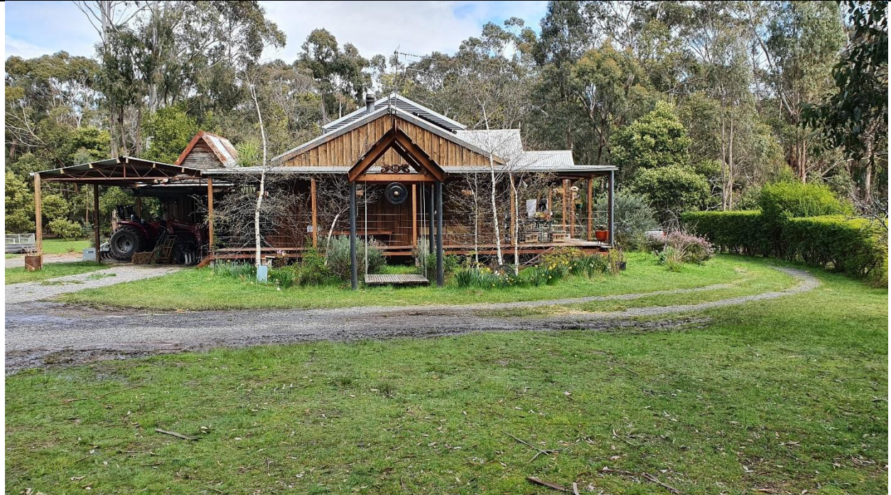
Photo 1 Looking south west to the dwelling in the central part of the site
