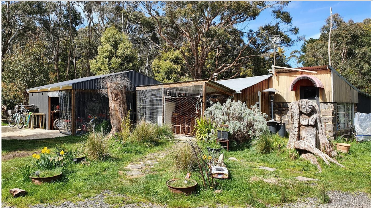
Photo 3 Looking south towards the existing outbuildings
