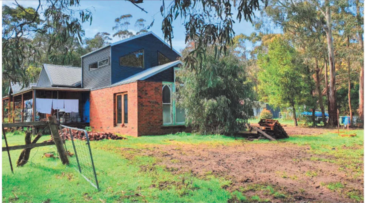
Photo 2 Looking south east to the existing dwelling
