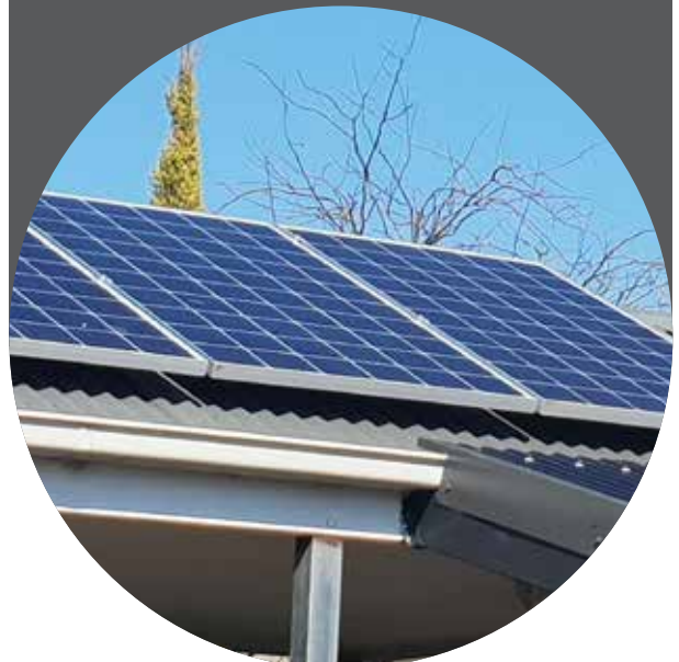
Solar panels installation
