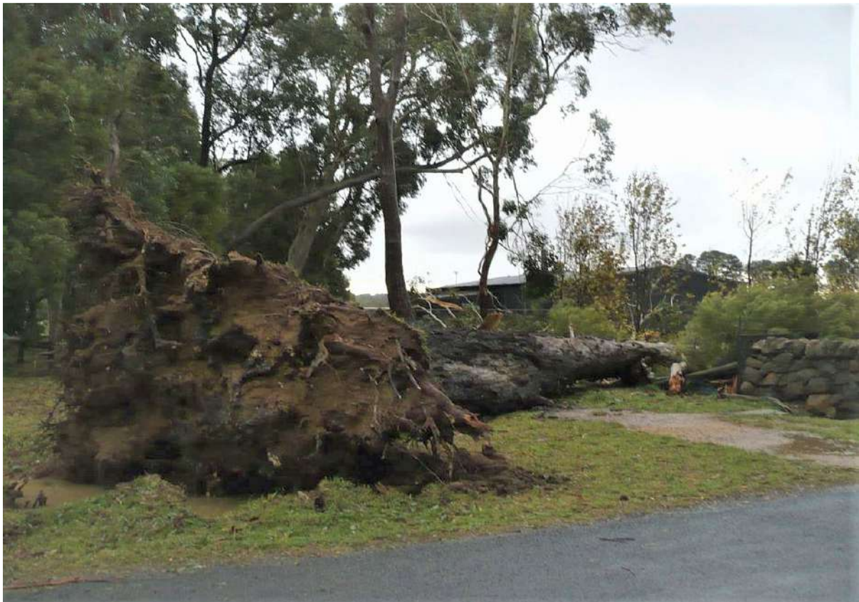
Tree at beginning of Gunyah Drive fell during storm June 2021 compromised by Culvert storm water 2.
