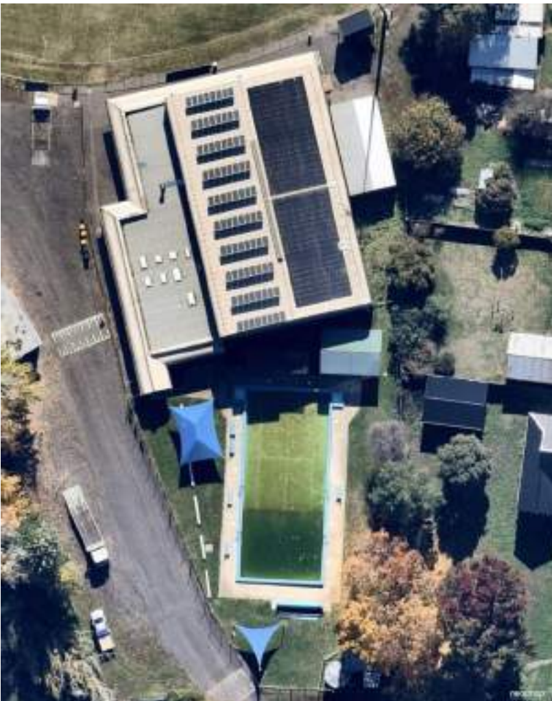
Figure 9: Aerial view of Clunes Outdoor Pool
