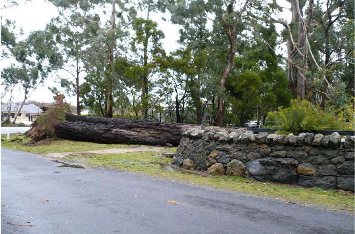
Tree at beginning of Gunyah Drive fell during storm June 2021 compromised by Culvert storm water.
