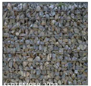
GABION RETAINING WALL
