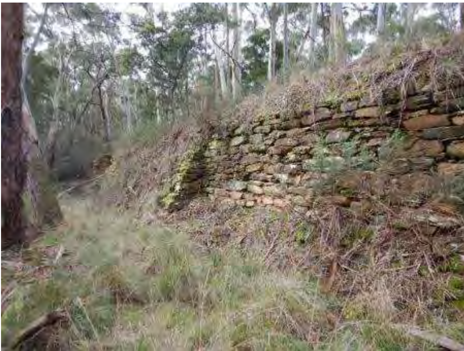
Photograph 16 Eatons Dam wall, Back Creek (Survey Unit 68)
