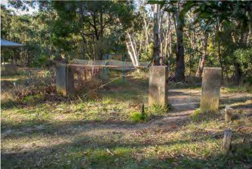
Photograph 37 Remnant gateposts and fence at Koala Park entrance.
