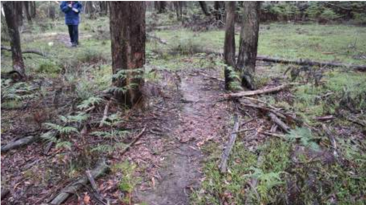
Figure 3 Example of existing trail close to trees with minimal excavation and minor compaction.
