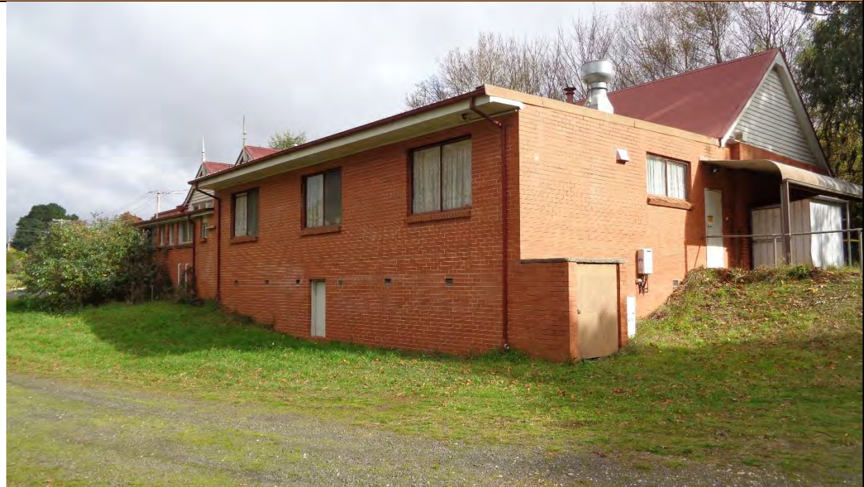
Photo 3 Looking south west to the existing building in the south west corner of the site
