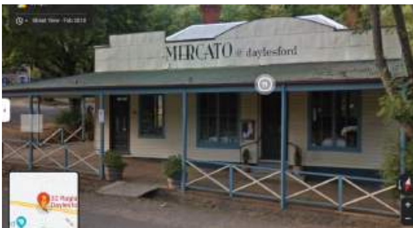
Figure 17 former Athens Hotel and Store - Raglan Street elevation (Source: Google Street View, February 2018)
