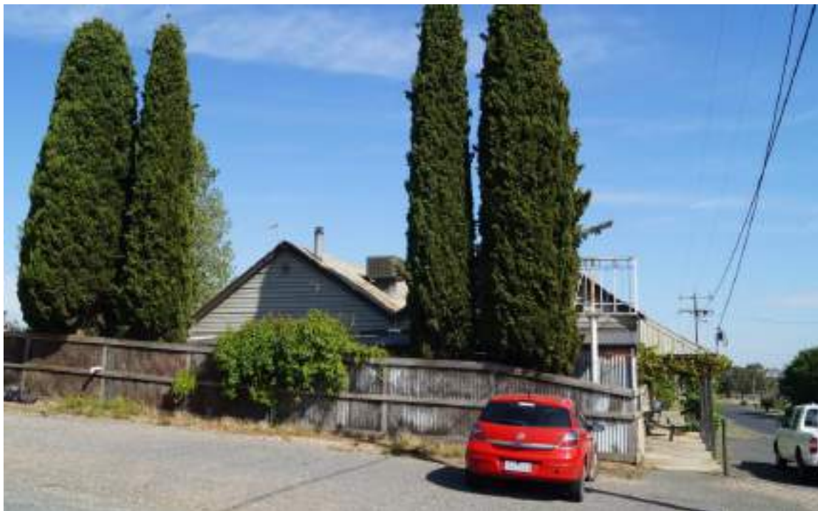
Figure 1 236 Main Road, Hepburn (Old Hepburn Hotel) - viewed from south, looking north (Source: Mandy Jean, Heritage Place Report 2020)
