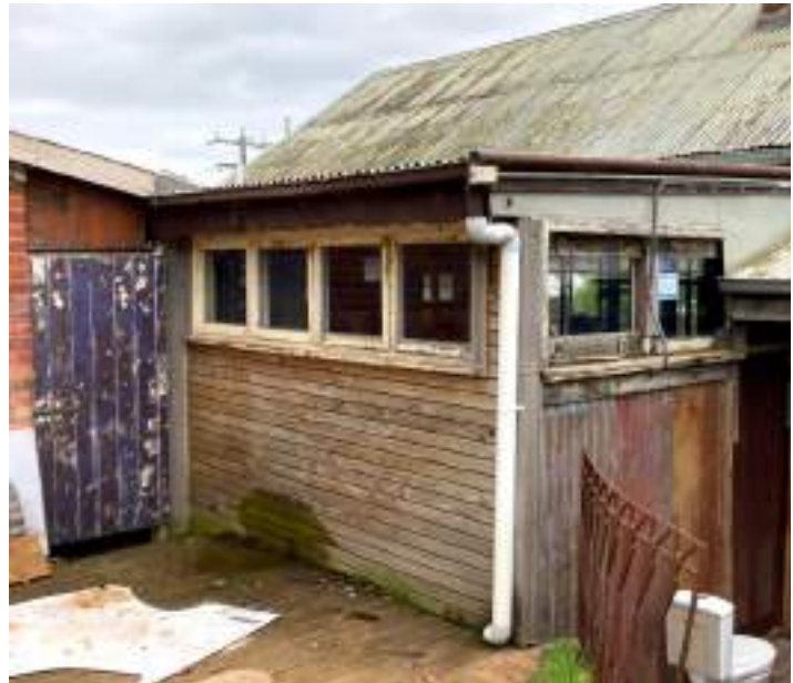
Figure 11 rear additions to building
