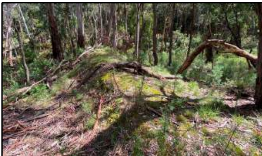
Figure 17: Section of earth dam embankment, Jackass Gully
