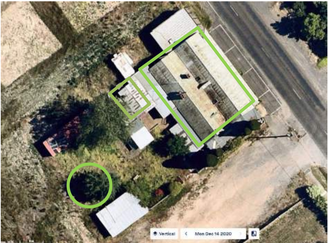
Figure 5 – 236 Main Road, Hepburn showing contributory elements of site as identified in Peer Review by Plan Heritage 2021
