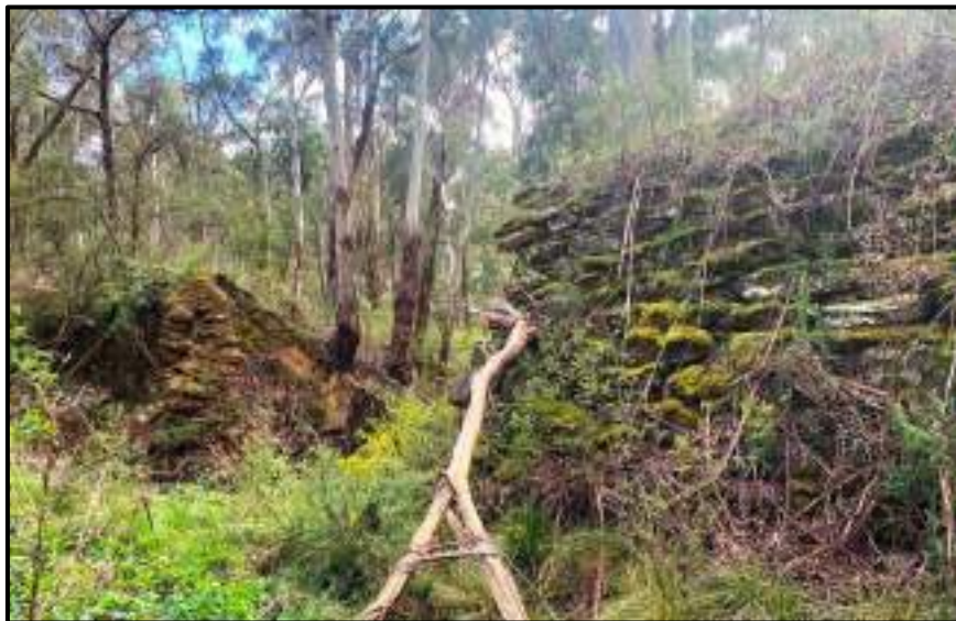
Figure 19: Exterior stone retained wall, Eaton's Dam
