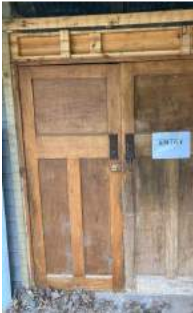
Figure 10 Internal doors repurposed at rear of building
