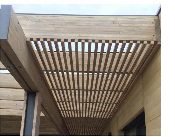
Timber Pergola stain finish & Steel Posts-paint finish charcoal
