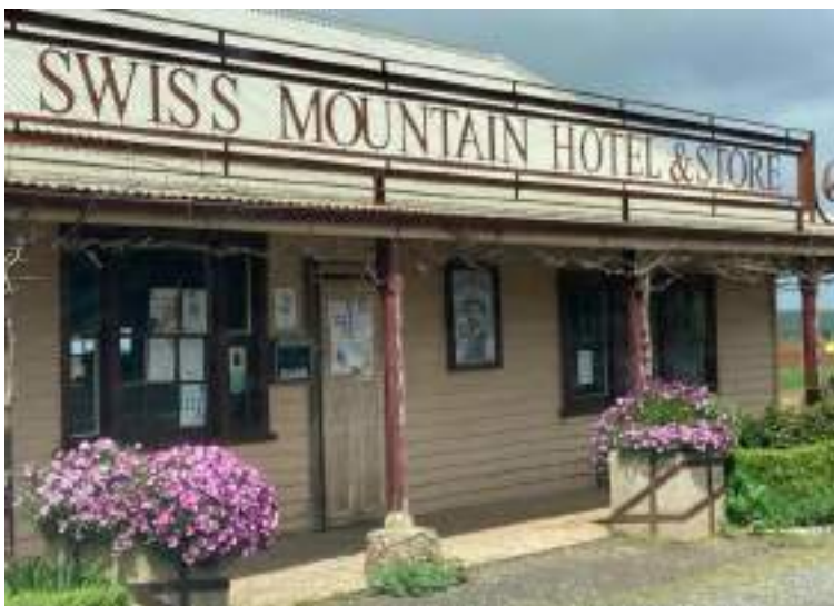
Figure 15 Facade -Swiss Mountain Hotel showing original façade
