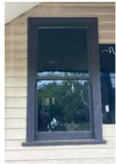
Figure 9 Example of original double hung timber sash windows on facade
