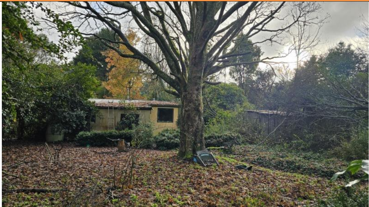
Photo 1 Looking north west to the existing house
