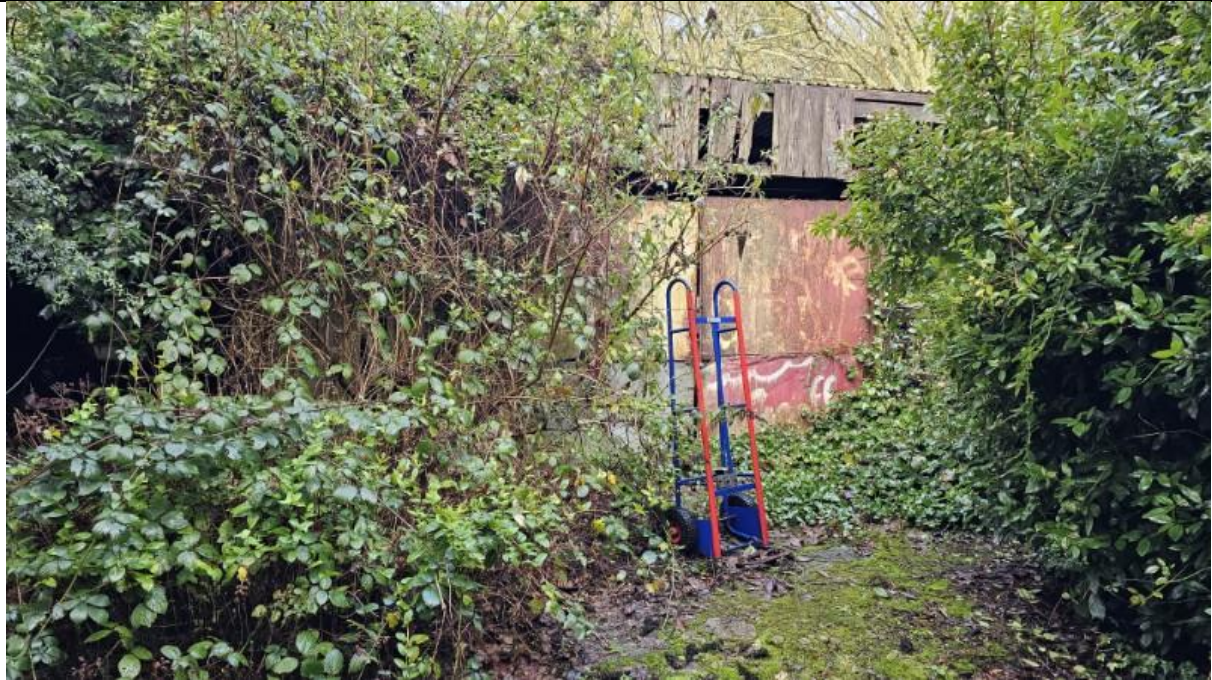
Photo 2 Looking south to an existing shed in the north west part of the site
