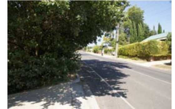
Figure 15: Lack of footpaths outside town centre
