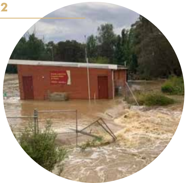
Flooding in Creswick after the storm event
