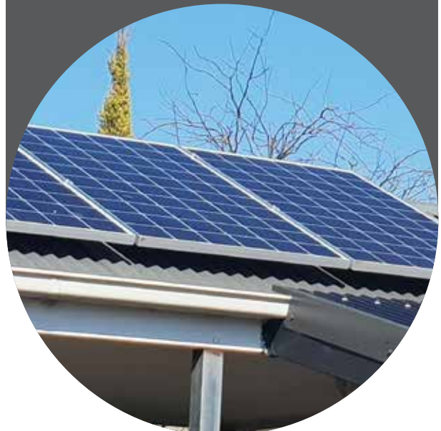
Solar panels installation
