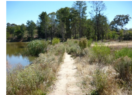
Walking track at Calembeen Park- damage has been sustained from floods in some places
