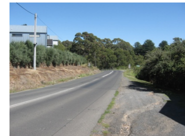
Area at Hepburn-Newstead Road where new footpath is required looking up toward Primary School.
