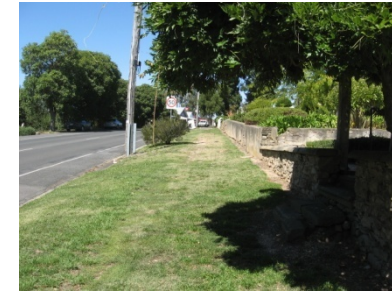
Looking back toward Hepburn along Hepburn Daylesford Road – footpath section missing.
