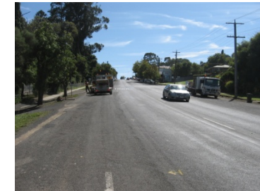
Vincent Street looking back to Daylesford. Daylesford Primary School on left and line marking shown partially removed.
