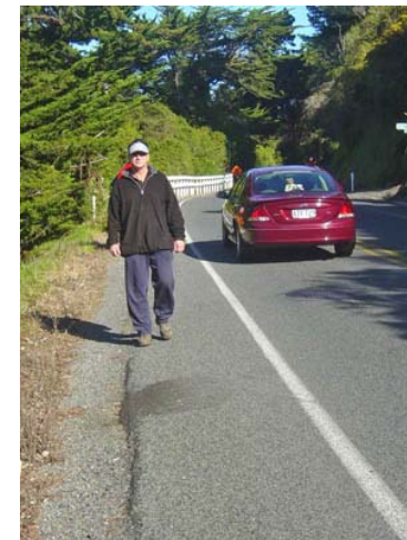
An example of sealing shoulders to provide space for cyclist and pedestrians
