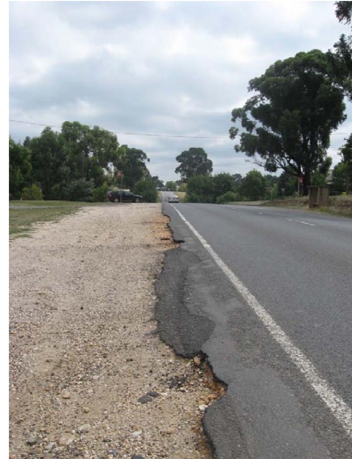
Road shoulder in Creswick North- Creswick –Clunes Road
