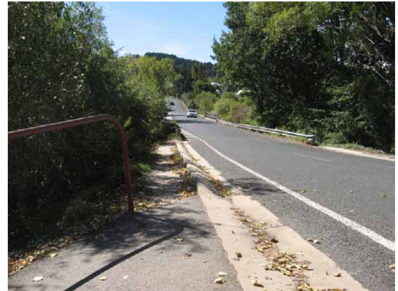
Current exit from Lake Daylesford on to Bleakely Street. Pedestrians are directed almost immediately on to the roadway.
