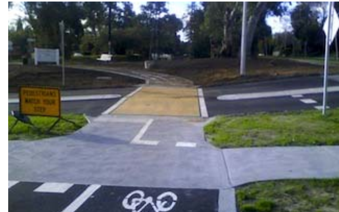
Trail crossing at road, prioritising the cyclist and walker
