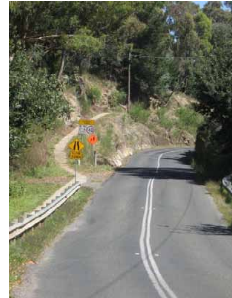
Pathway to Hepburn Primary School is steep and requires some railing to protect from the edge of the incline.
